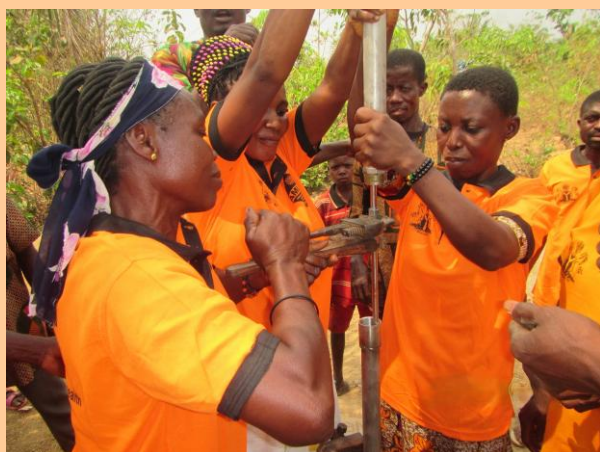
Women WASHCOM members installing the borehole at Azu-Akpalolo, Izzi L.G.A.
