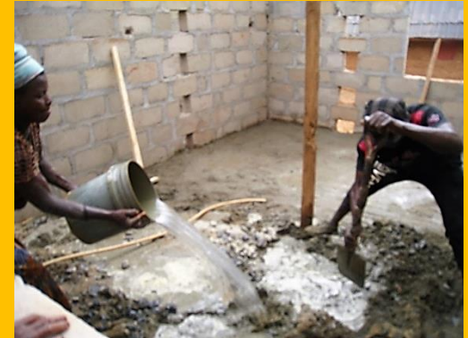
Community members working on construction at Uloanwu Health Center
