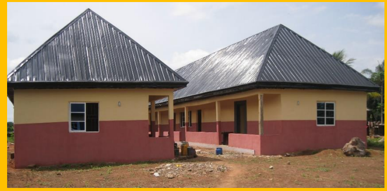
The Ohagelode Staff quarter provides 10 self-contained units for staff close to the health center
