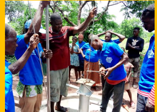
WASHCOM installing new borehole at Ndiegu Azu, Amana, Ezza South LGA
