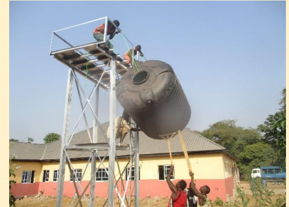
Water tower ready for Ohagelode completion
