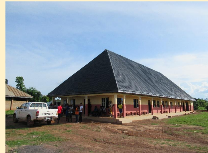
The main hospital building at Uloanwu
