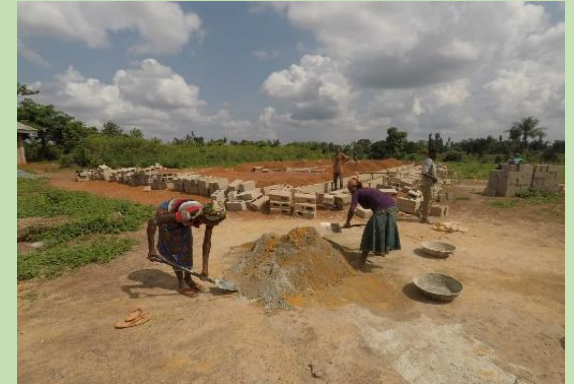
Construction starts on main clinic building
