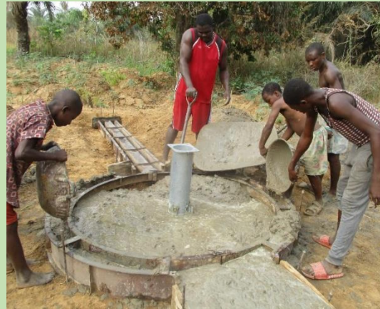
Platforming at new borehole in Obeagu, Isu
