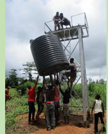
Raising the water tank
