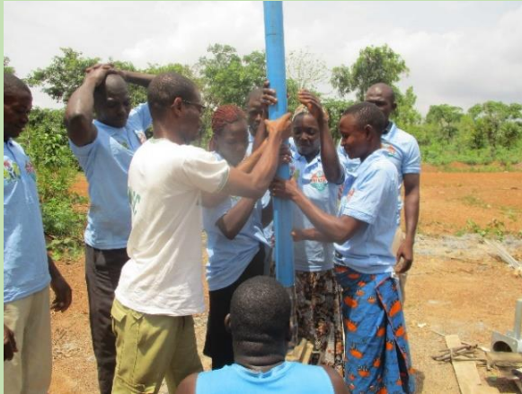
Agharaoza installation of new borehole
